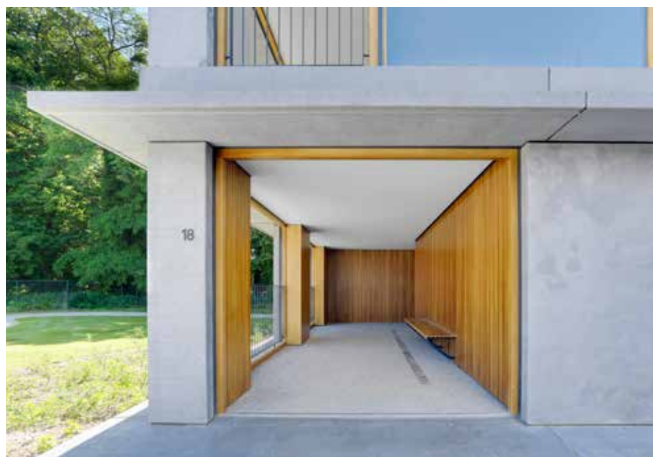
BMT Parkvilla Boechout © Bart Gosselin
